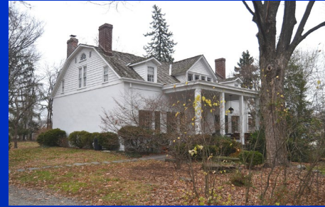
Martin Berry House Rehabilitation Location: Township of Pequannock Grant: $626,560 (2018, 2019 Grants)
