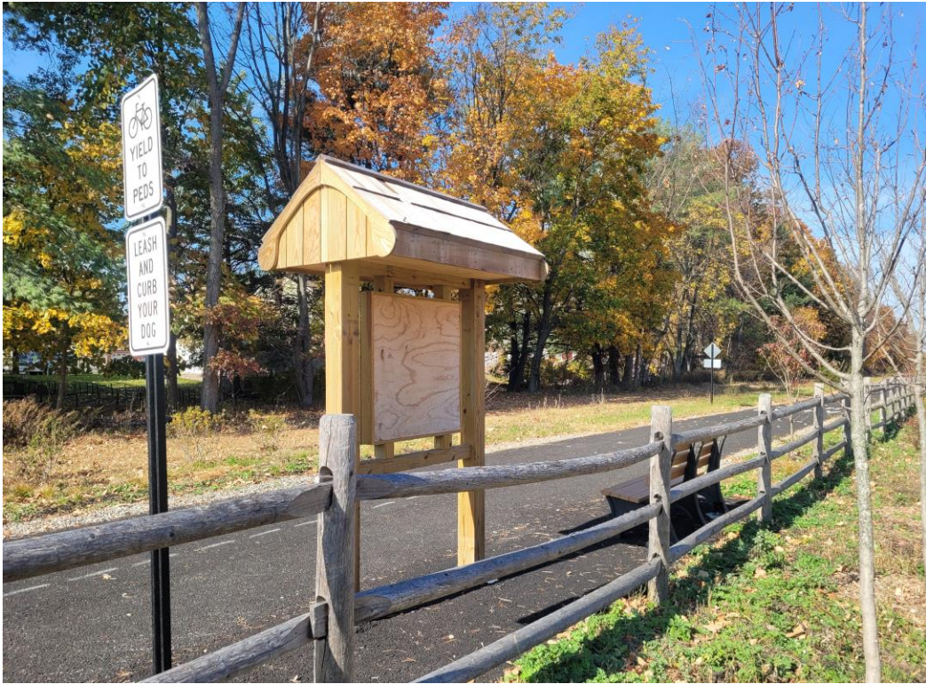
The 4.8-mile Pompton Valley Rail Trail will be completed and fully open Spring 2025.
