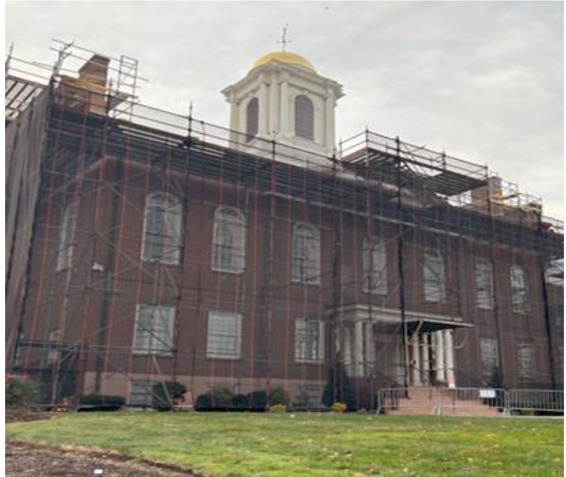
The historic Morris County Courthouse is undergoing brickwork and restoration.
