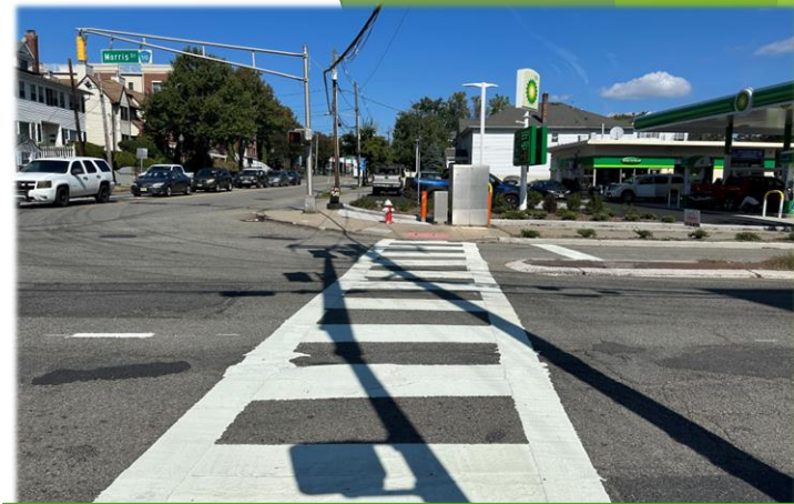
East crosswalk at Morris Street and Ridgedale Avenue
