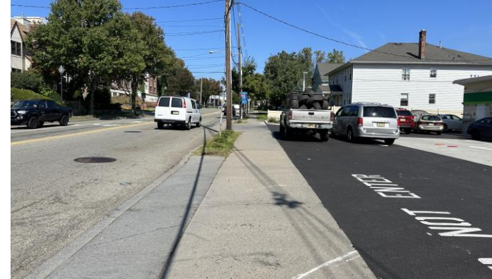
Non-compliant sidewalk across driveway aprons
